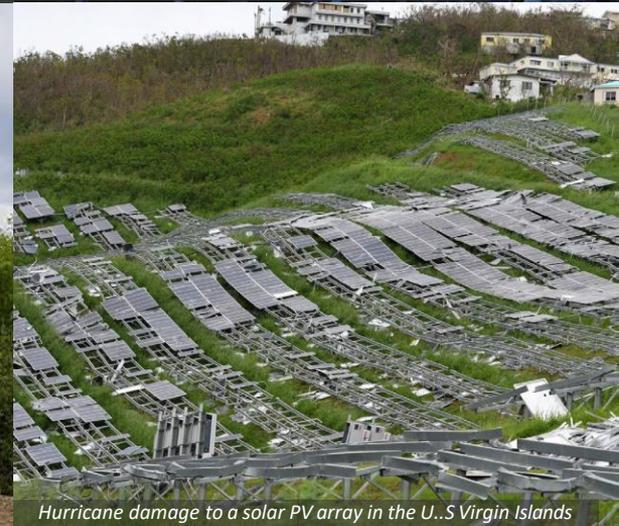
*Hurricane damage to a solar PV array in the U.S Virgin Islands*
