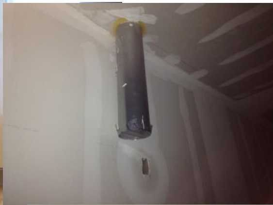
Exhaust fan ducts
