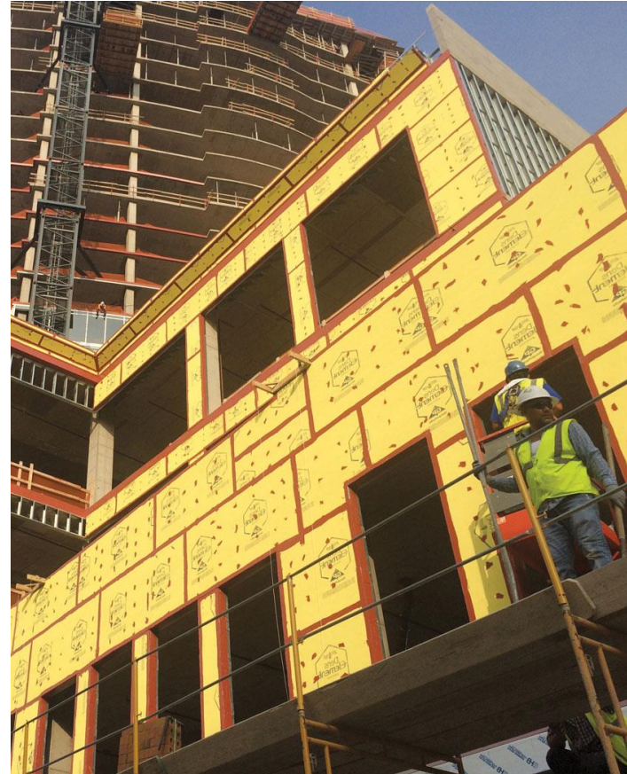
Photo courtesy of U.S. Gypsum
