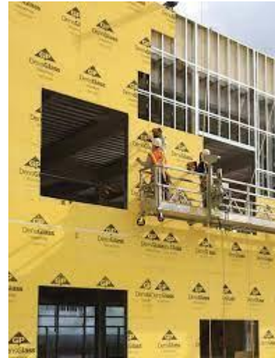
Steel Stud/Exterior Sheathing
