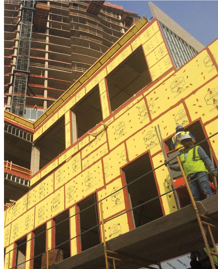
Photo courtesy of U.S. Gypsum
