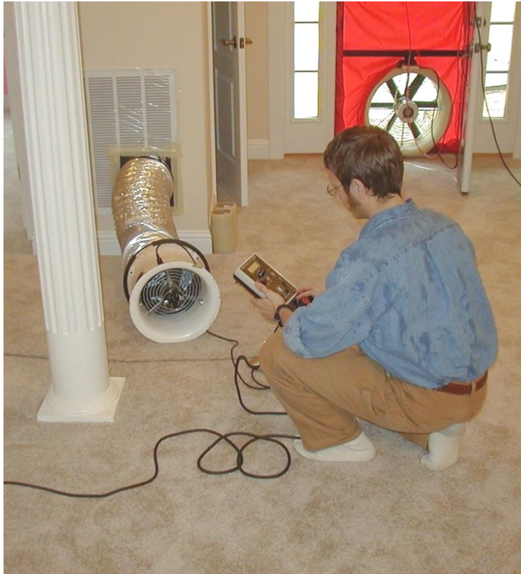
Pressurizing the system; connected at the largest return
