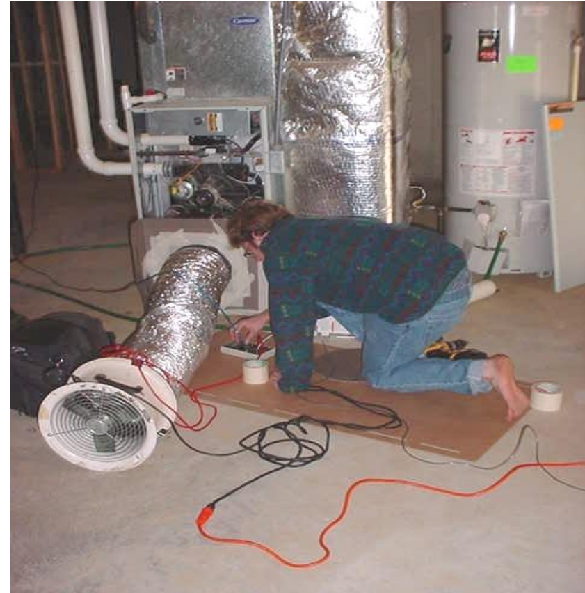
Depressurizing the system; connected at the air handling unit
