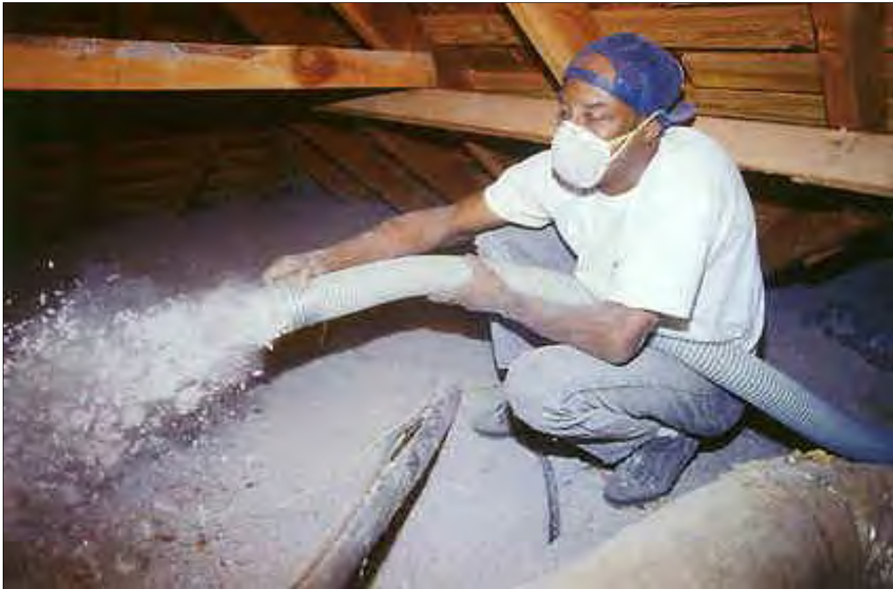
Loose fill insulation (typically fiberglass or cellulose)
