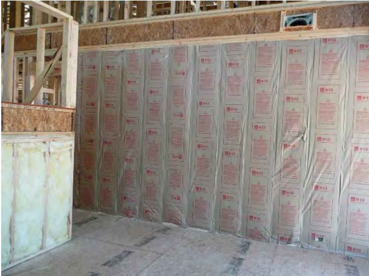
Kraft-faced fiberglass batt insulation
