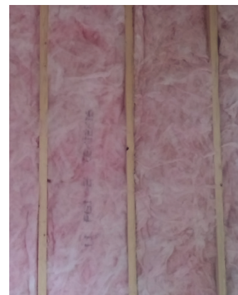
Insulation in full contact with all six sides of stud cavity
