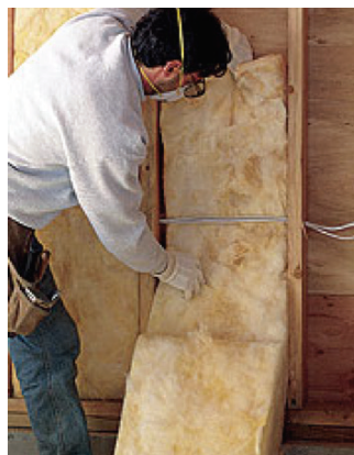
Insulation is cut and split around electrical wiring
