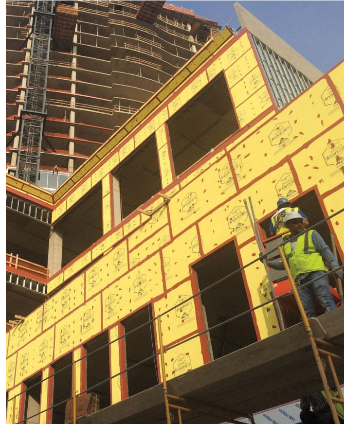
Photo courtesy of U.S. Gypsum
