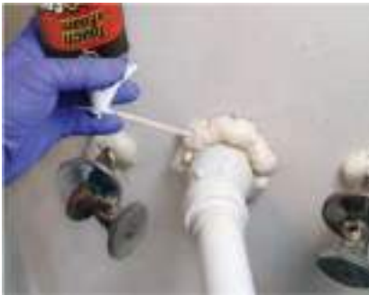
Seal plumbing penetrations
