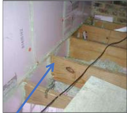
Install Knee wall blocking
