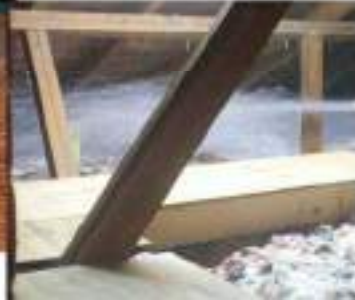
Energy Truss with full height insulation (recommended)
