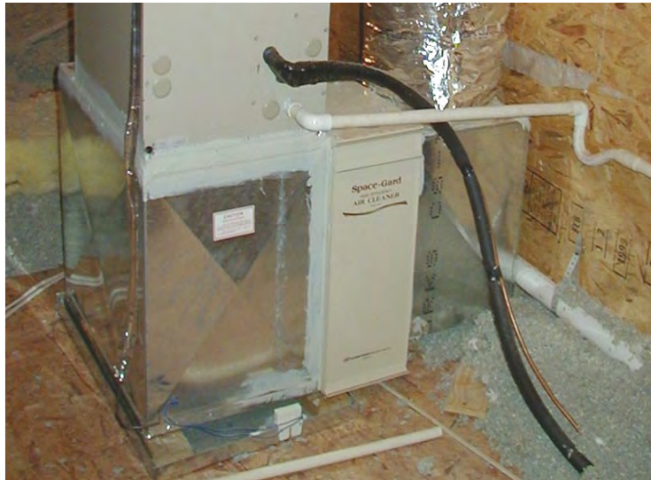
"Filter Lock" uses magnets to seal access
