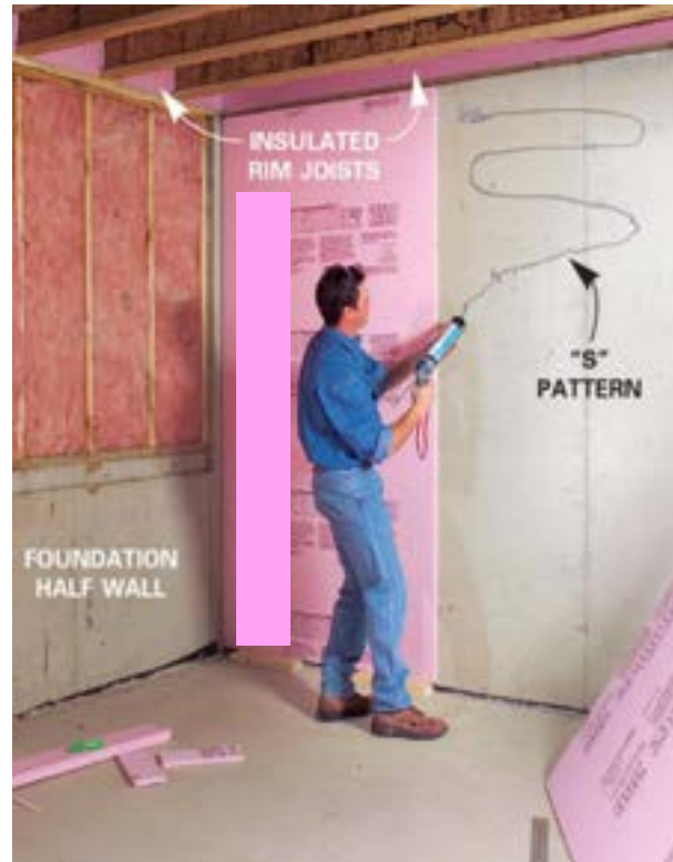
Foam board on concrete
