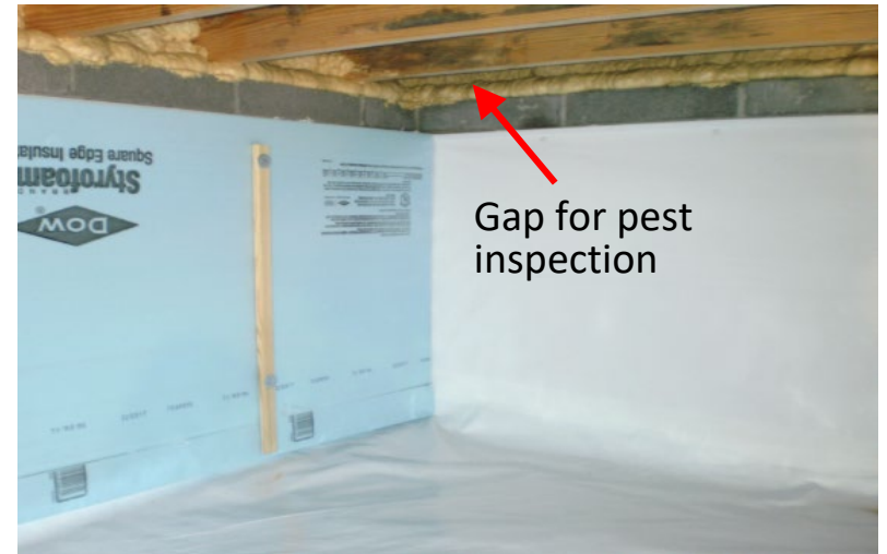
SF suggestion: taped, hinged "plug" of rigid insulation board in gap
