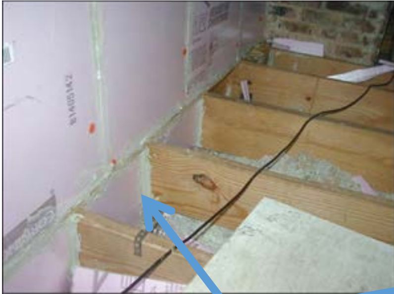
Install Kneewall Blocking
