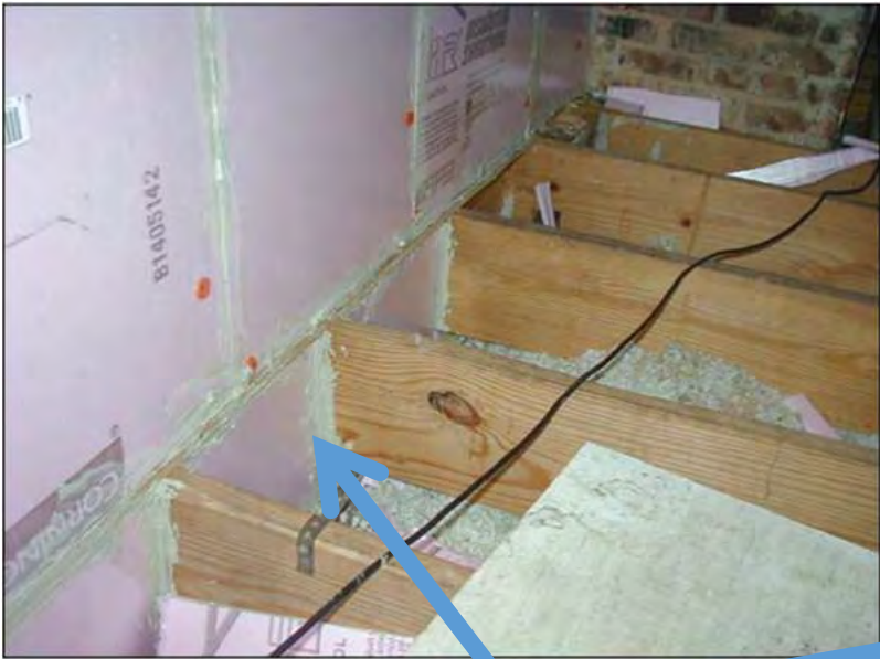
Install Kneewall Blocking
