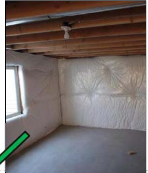
Fiberglass batt w/ vinyl backing
