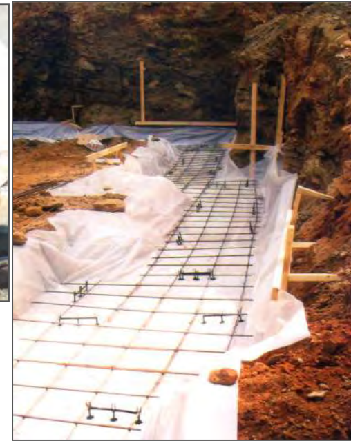
Plastic wrapped beneath footing
