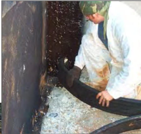
Plastic wrapped beneath footing
