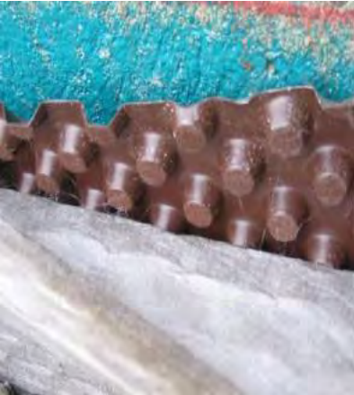
Spray on waterproofing plus drainage board
