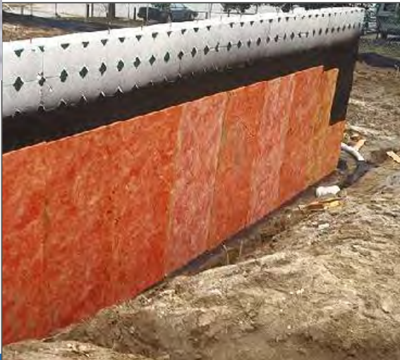
Spray on waterproofing plus drainage board
