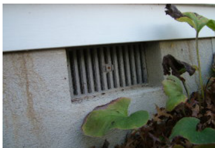
Crawl space vent
