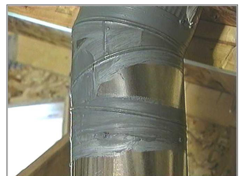
This duct has been sealed but not insulated 2
