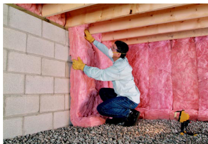
Proper installation (no vent)
