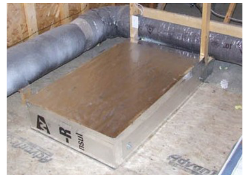
Insulated attic hatch and insulated ducts 1
