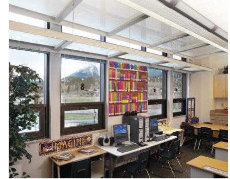
More Efficient Lighting System
