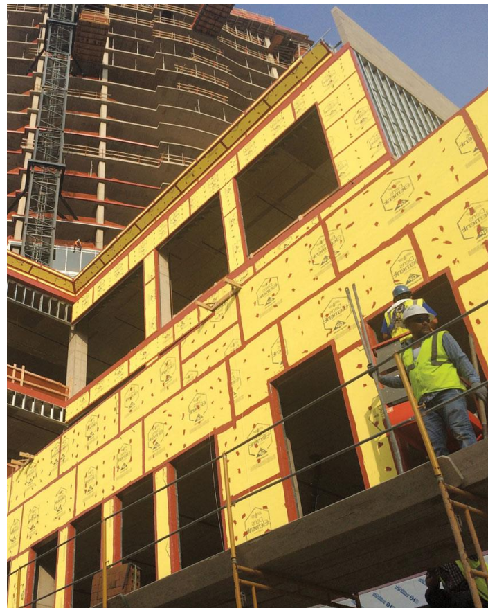
Photo courtesy of U.S. Gypsum
