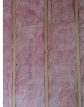
Insulation in full contact with conditioned space
