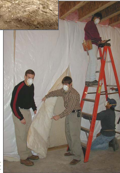
Fiberglass blanket, ~R-3.5+/inch
