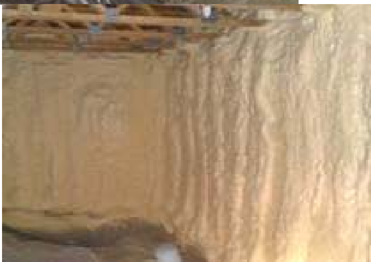
Closed Cell Foam, ~R-6+/inch
