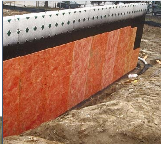
Rigid Fiberglass board, ~R-3.5/inch
